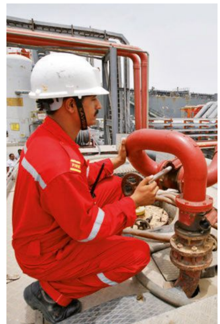
Turning on the loan pipe
